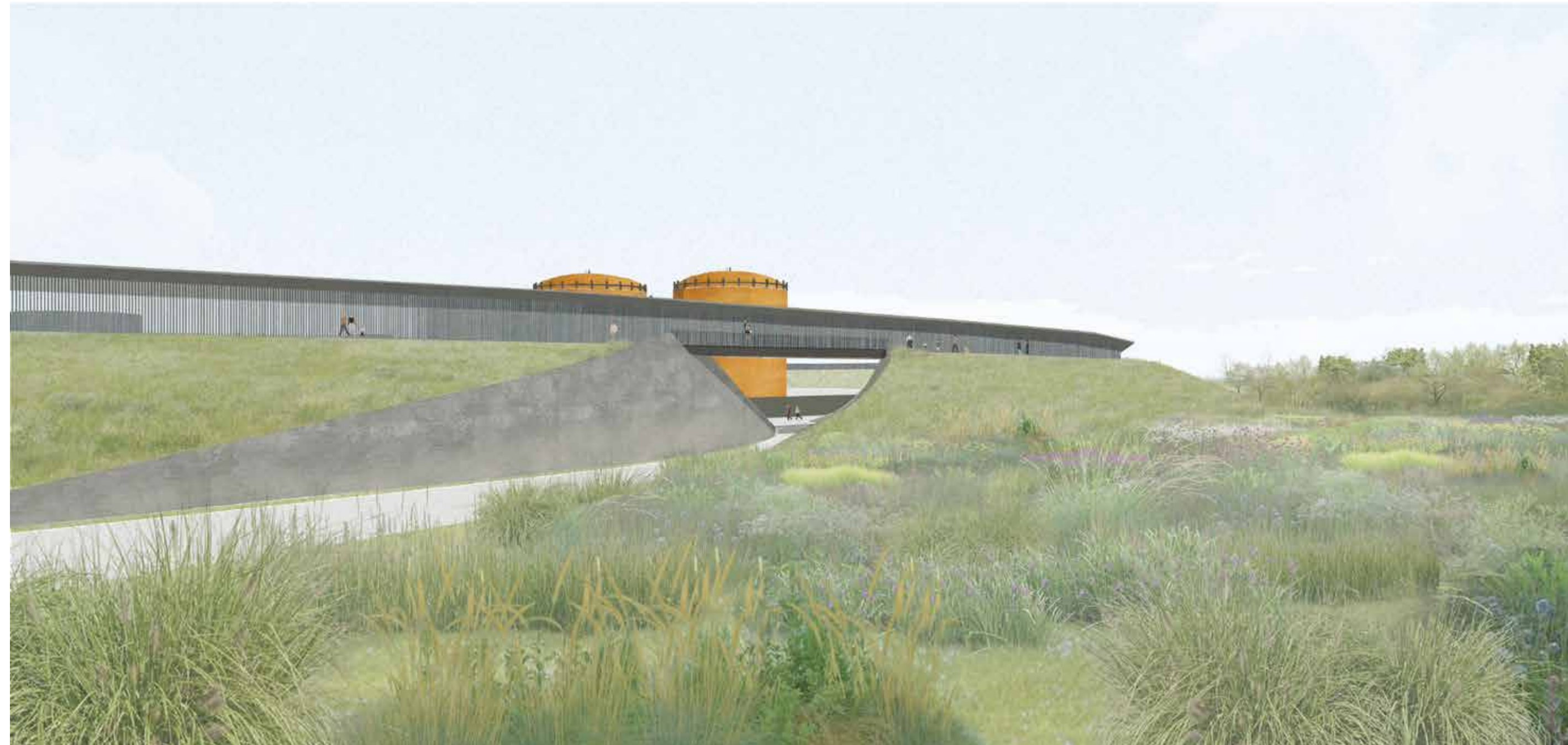
Illustrative visualisation of the anaerobic digester cladding with a more contrasting finish behind additional screening on top of the earthwork bank
